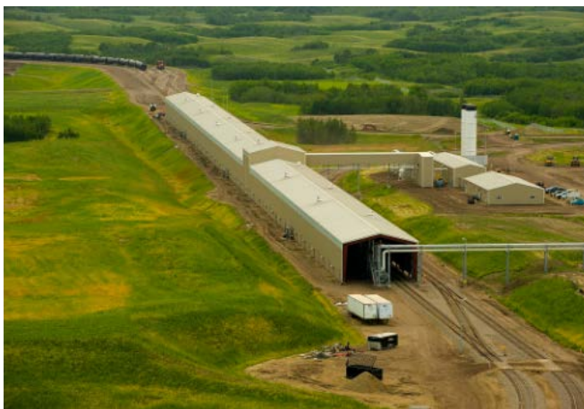
Hardisty Rail Terminal
